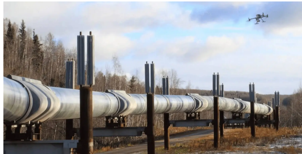
Fig. 3 Pipeline Inspection. Image courtesy of Flytbase[10].
