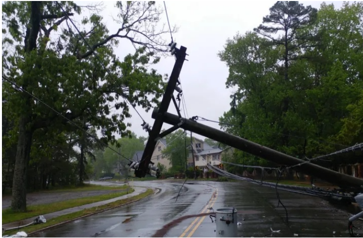
Fig. 1 Downed power line in rainy weather
