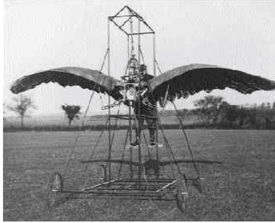
Fig. 2 E.P. Frost's 1902 Internal Combustion Ornithopter [11]
